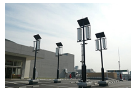
Windmills and solar panels
