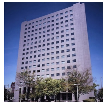
Hankyu Corporation Head Office Building
