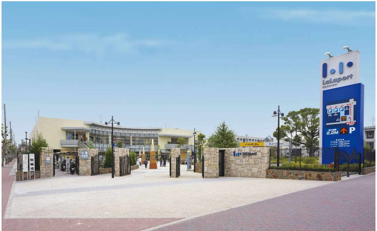
Photograph of External Facade of LaLaport KOSHIEN(site)
