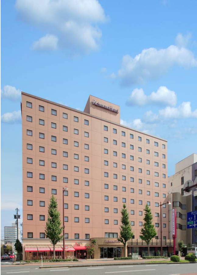
Photograph of External Facade of Richmond Hotel Hamamatsu
