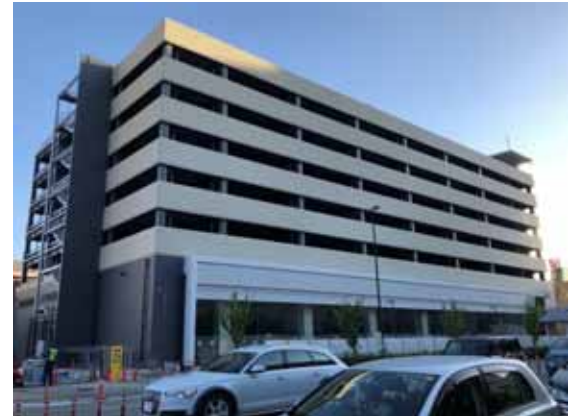
As of the end of June 2018 (Photographed from north side)
