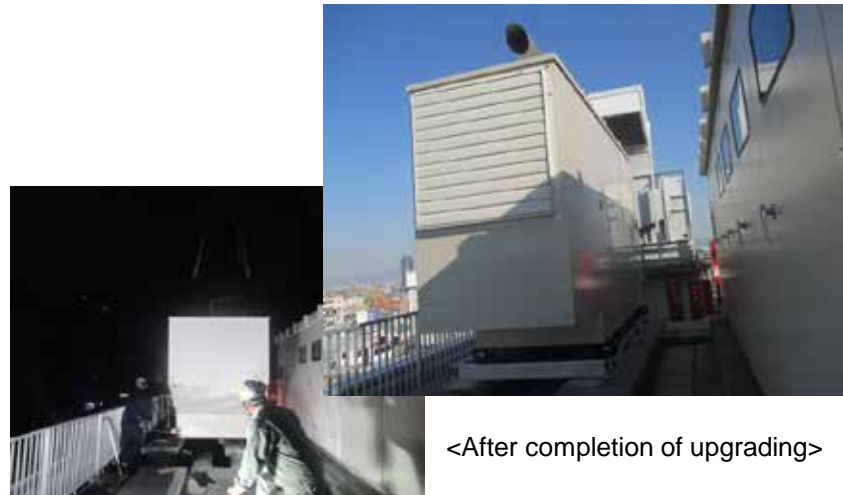
<Removal of old power generator>
