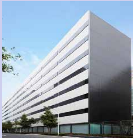
Shiodome East Side Building
