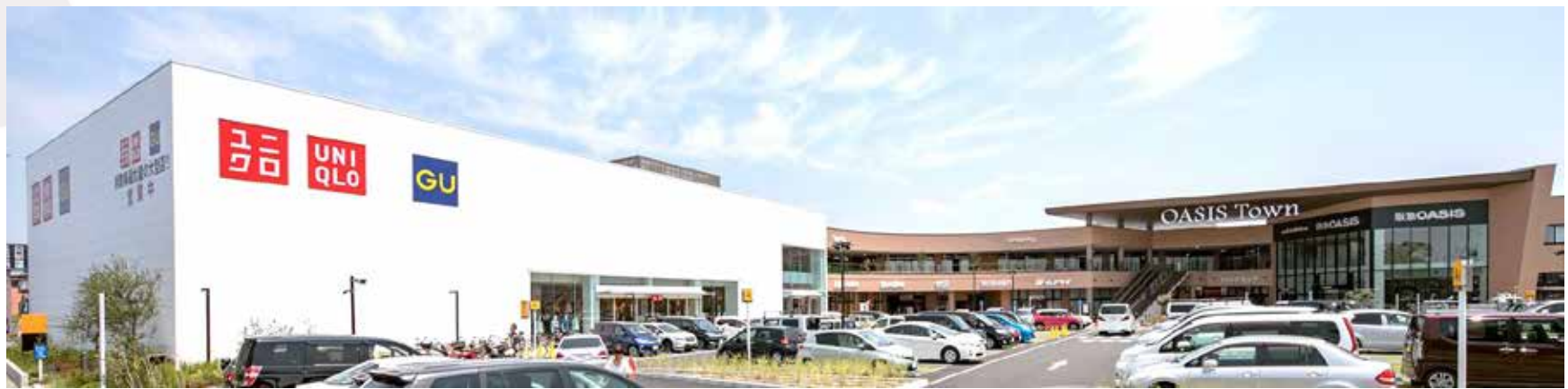
External view of the facility
