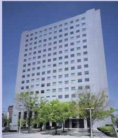
Hankyu Corporation Head Office Building
