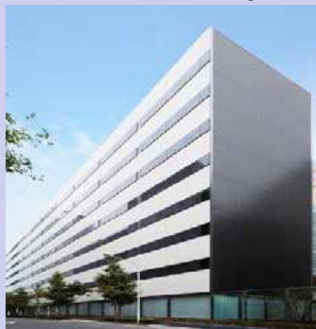
Shiodome East Side Building
