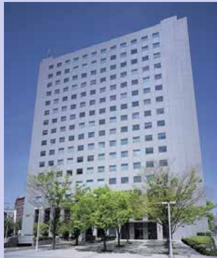
Hankyu Corporation Head Office Building
