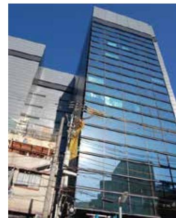
Implemented repair work on exterior walls in 3 phases. In this phase, implemented repair of window seals, painting of wall surfaces, etc. on the south-facing and west-facing exterior walls.
