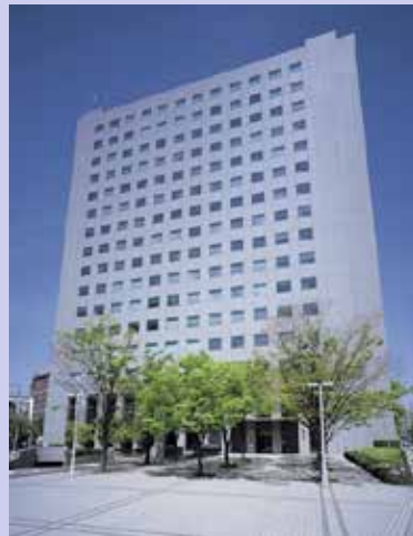
Hankyu Corporation Head Office Building
