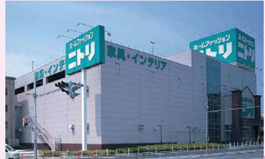
Nitori Ibaraki-Kita Store (Site)
