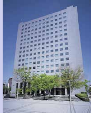
Hankyu Corporation Head Office Building
