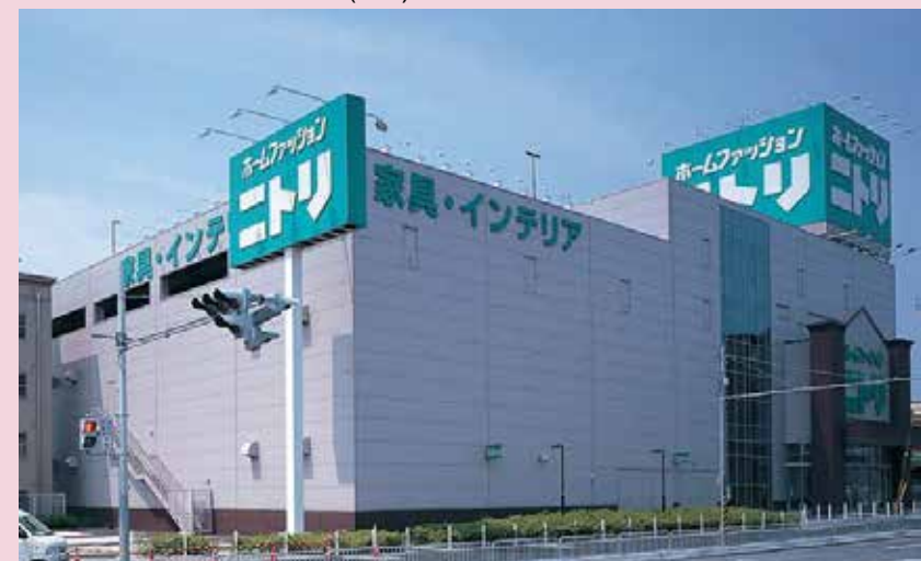
Nitori Ibaraki-Kita Store (site)
