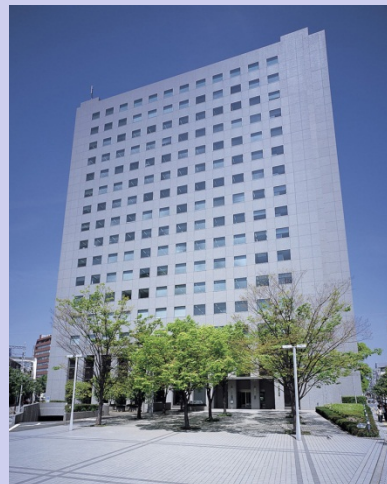
Hankyu Corporation Head Office Building
