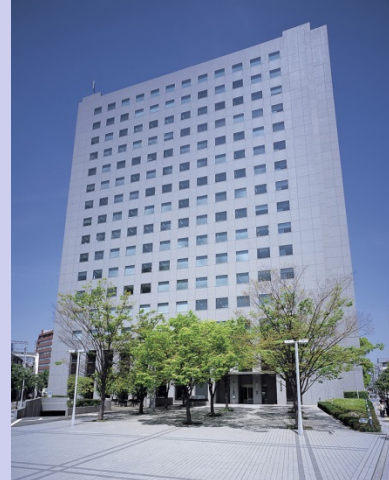
Hankyu Corporation Head Office Building
