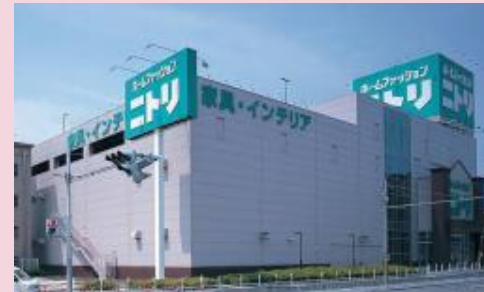
Nitori Ibaraki-Kita Store (Site)
