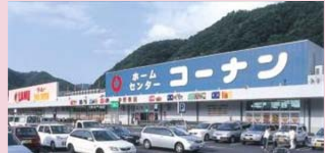
Kohnan Hiroshima Nakano-Higashi Store (Site)
