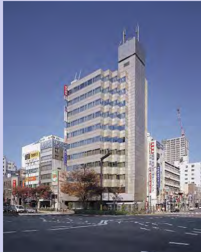
Ueroku F Building
