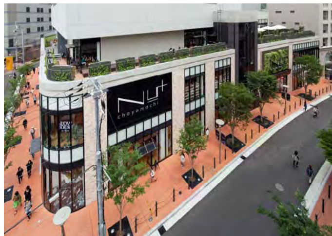
NU chayamachi Plus which opened in April
