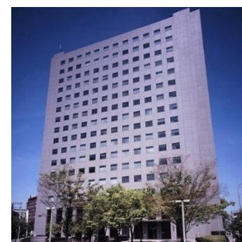
Hankyu Corporation Head Office Building
