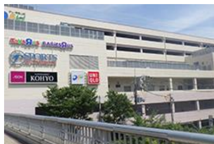
Repairing the exterior wall at Dew Hankyu Yamada
