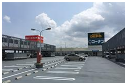
Waterproofing work on the roof of Takatsuki-Josai Shopping Center
