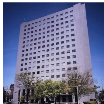
Hankyu Corporation Head Office Building
