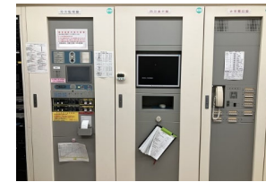
Repair work on fire protection control equipment at Kitano Hankyu Building
