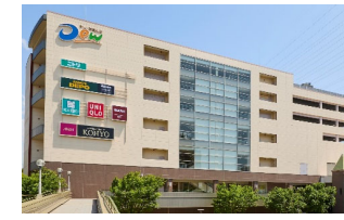
Repairing the exterior wall at Dew Hankyu Yamada
